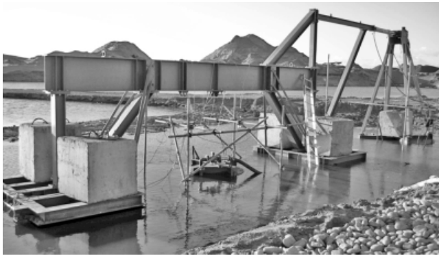
Fig. 5. Test rig showing the 1.5 m caisson installed in foreground and 3.0 m caisson in background after a jacking test had been completed
